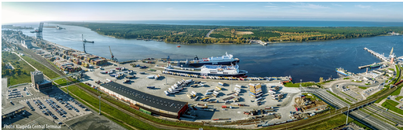
Photo: Klaipėda Central Terminal
