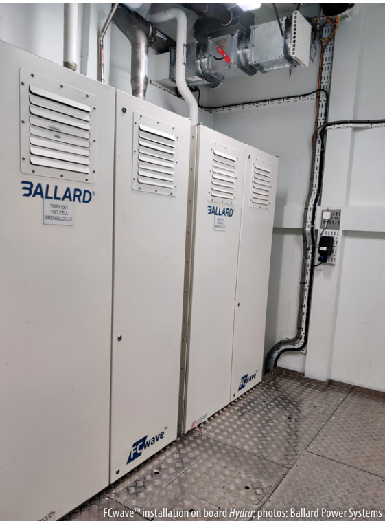
FCwave™ installation on board Hydra; photos: Ballard Power Systems
